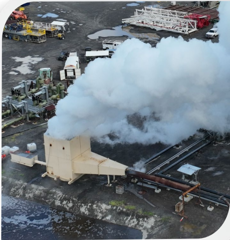
KS-22 Flow Test
